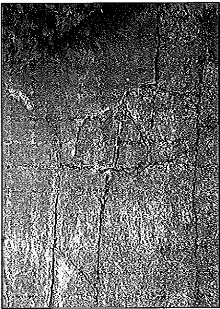
Photo 4: Cracked driveway.
